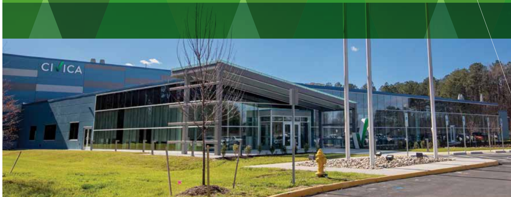
Civica's Petersburg, VA manufacturing facility.
